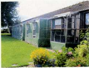
IPC BELGIUM Loft
